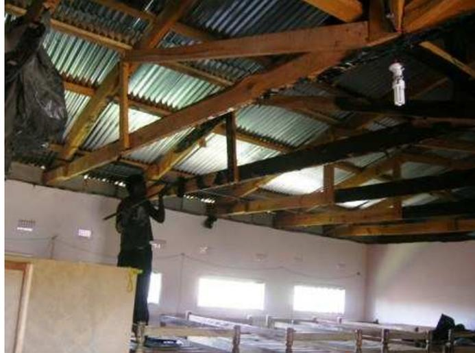
Ceiling beams being painted with white ant protector. No while ants in beams, but the reed ceiling mats had to be removed as they were infested with white ants.
